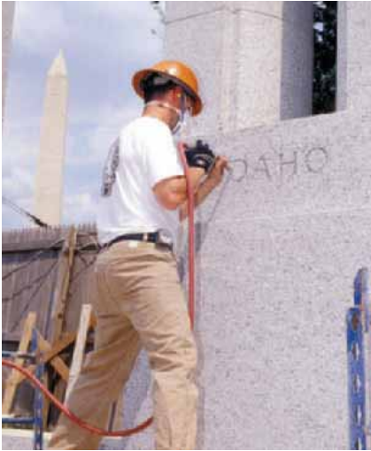
Completing the stonework at World War II Memorial
