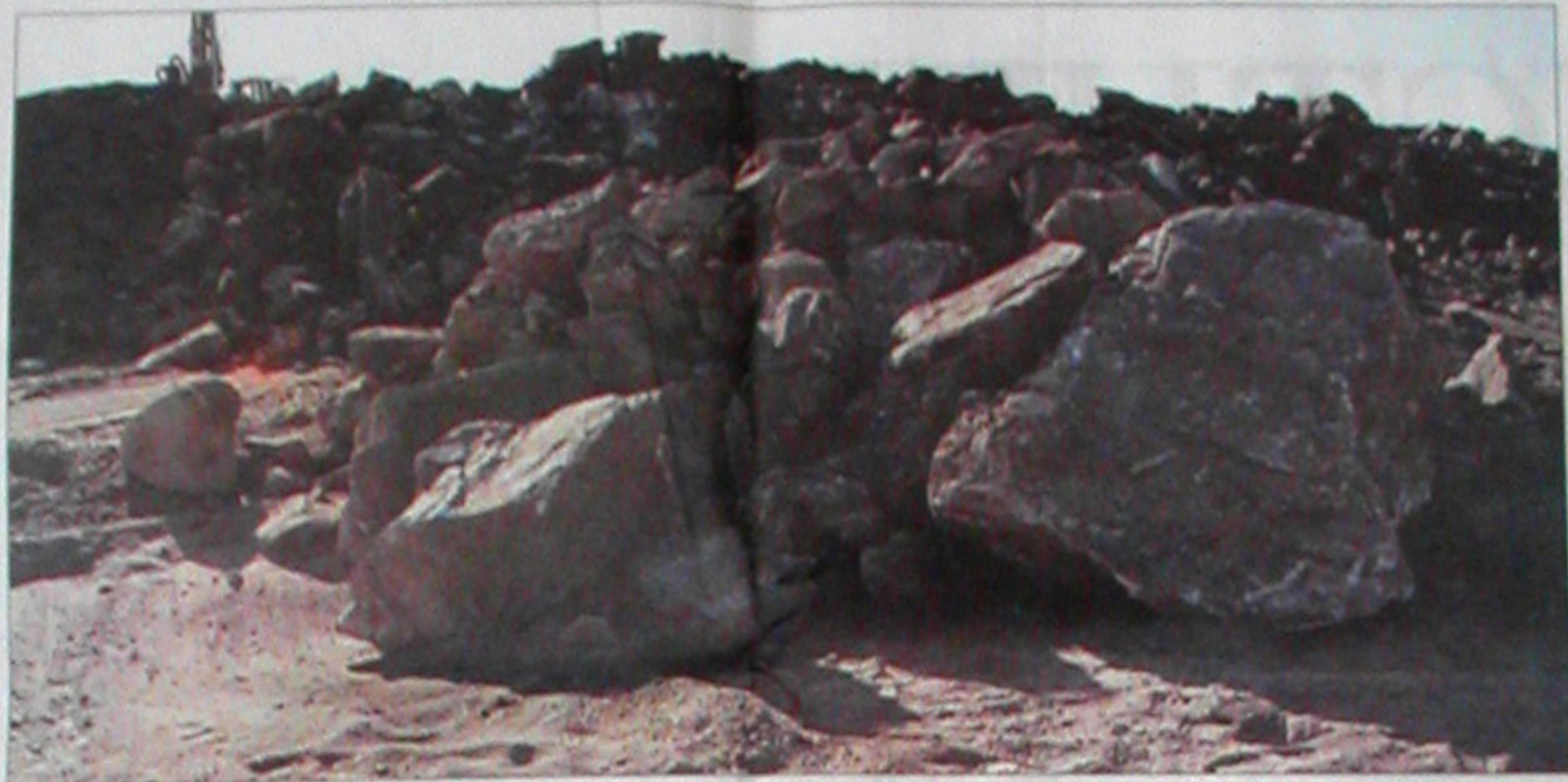
ROCK AND ROLL: The aftermath of the blast leaves a pile of boulders to be moved elsewhere on site. A backhoe fitted with a special ramming device breaks the boulders into smaller rocks.
