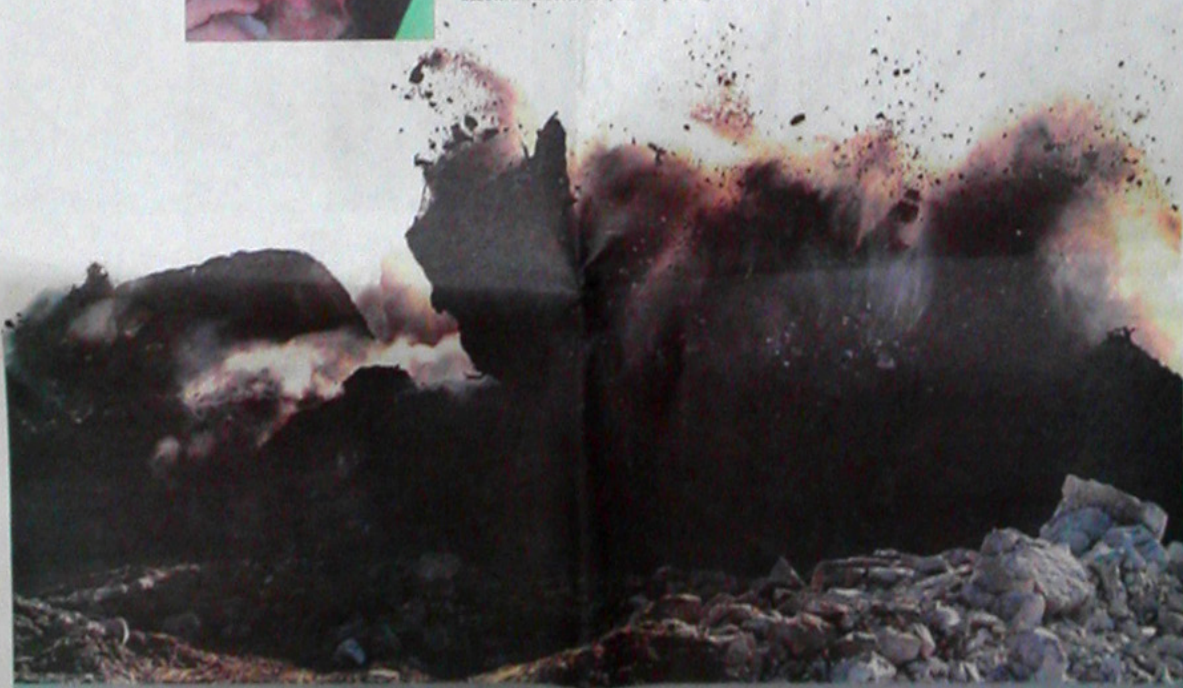
BELOW: Dirt and boulders fly into the air during the blast.
