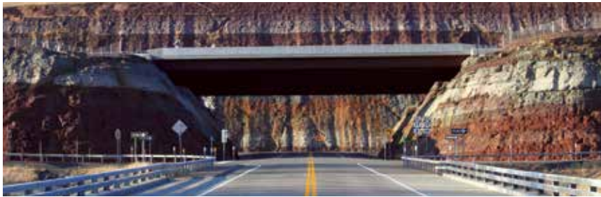
MD&B designed and produced the radius pre-split intersections, leaving a stable, eye-catching rock intersection.
