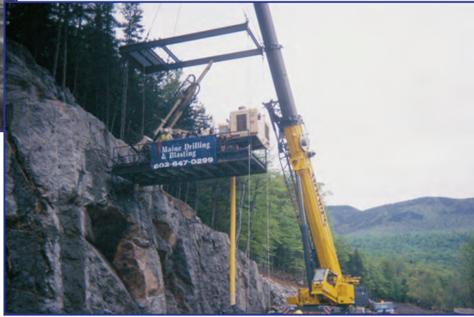
Installing rock bolts is another specialty of MD&B.
