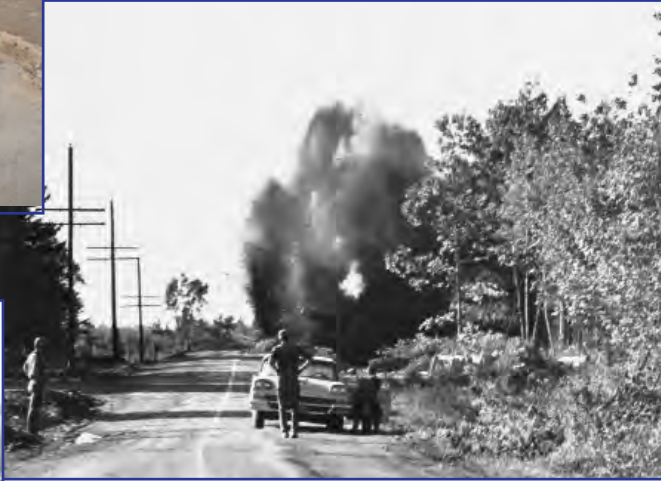
In the early days, blasting was hardly the sophisticated science that it is today.
