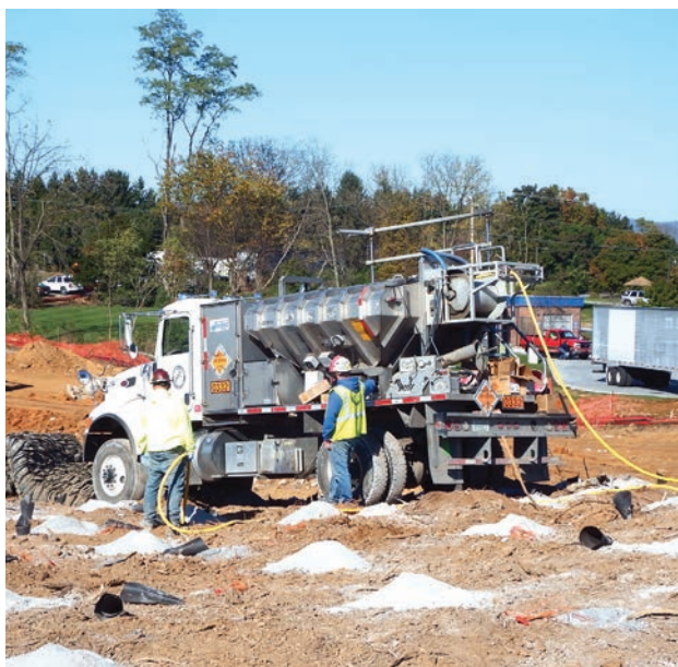
The Independent Explosives crew fills boreholes with blasting material in preparation of the upcoming blast.
