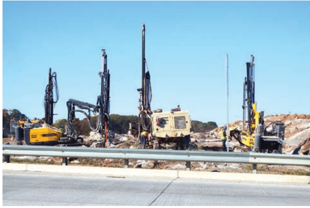
Drillers are busy boring blast holes for an upcoming detonation.
