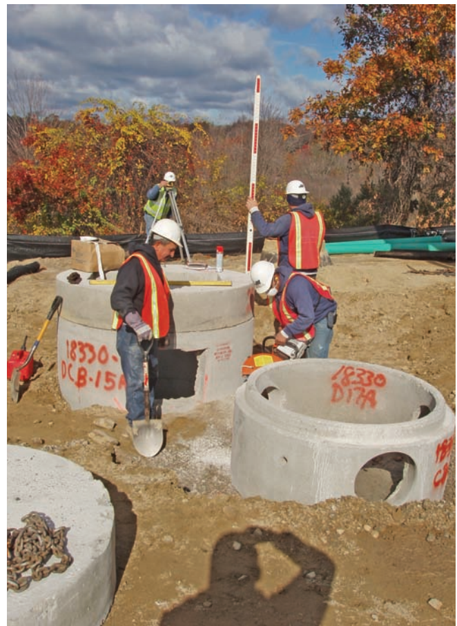
Masterson crew works on utility system manholes.
