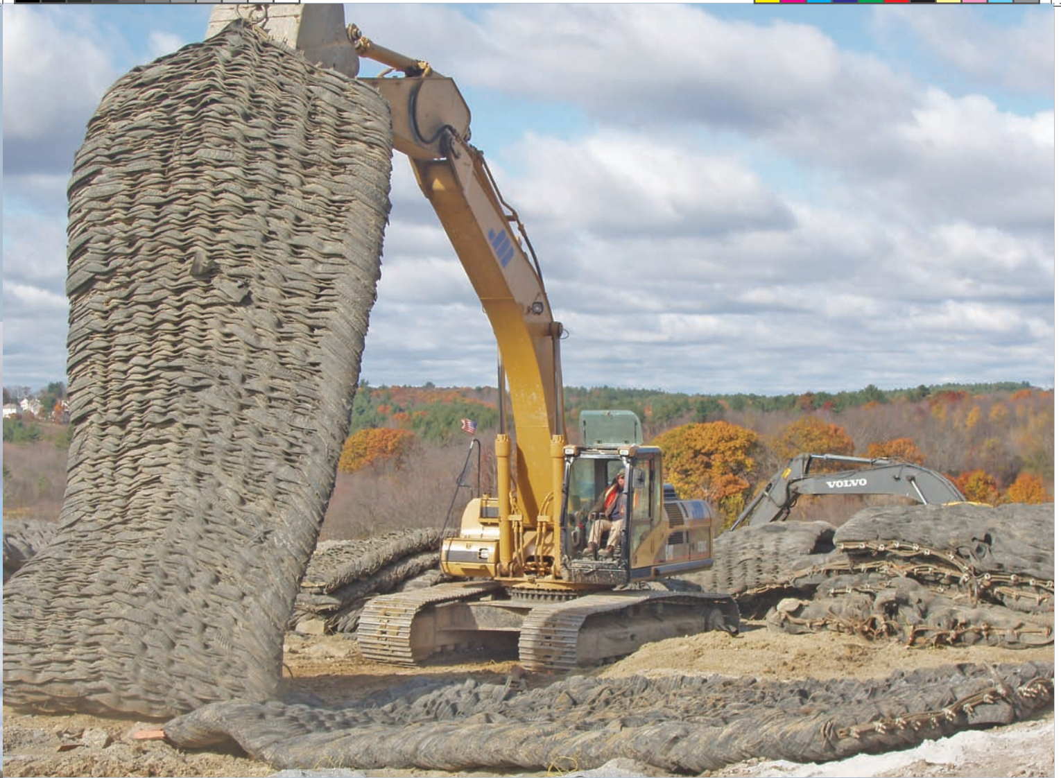
Above: CAT 330C excavator moves a blasting mat to cover the next shot. Below: A Volvo excavator loads blasted rock into a CAT articulated off-highway truck.
