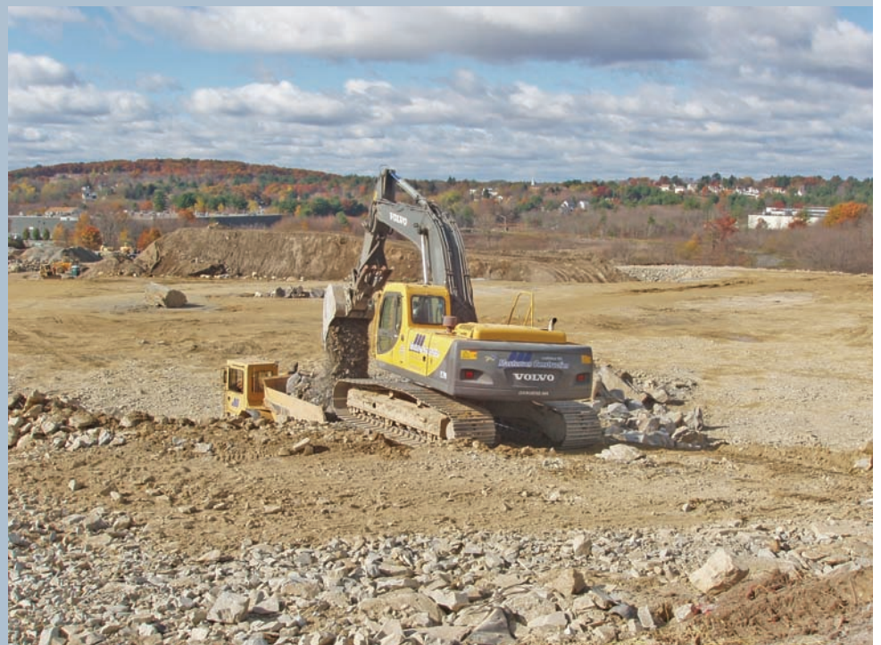
Above: CAT 330C excavator moves a blasting mat to cover the next shot. Below: A Volvo excavator loads blasted rock into a CAT articulated off-highway truck.
