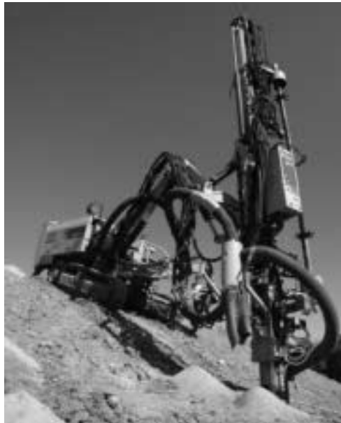
Atlas Copco hydraulic drill at Rockland. Maine Drilling & Blasting photo.
