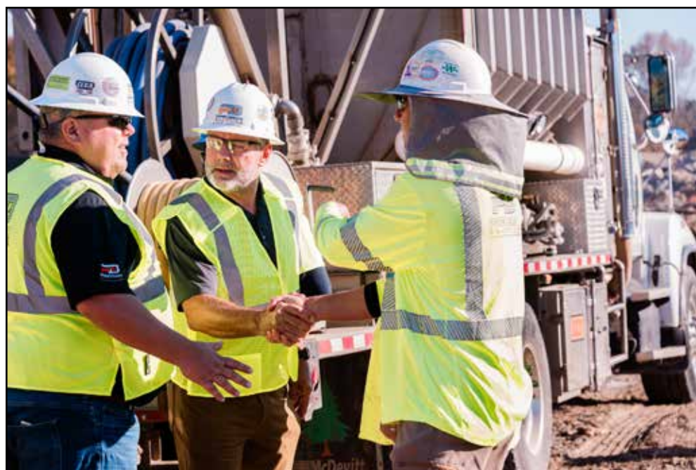
■ The Precision Blasting crew works together on the Villa Rica North Loop Bypass job site in Georgia.
