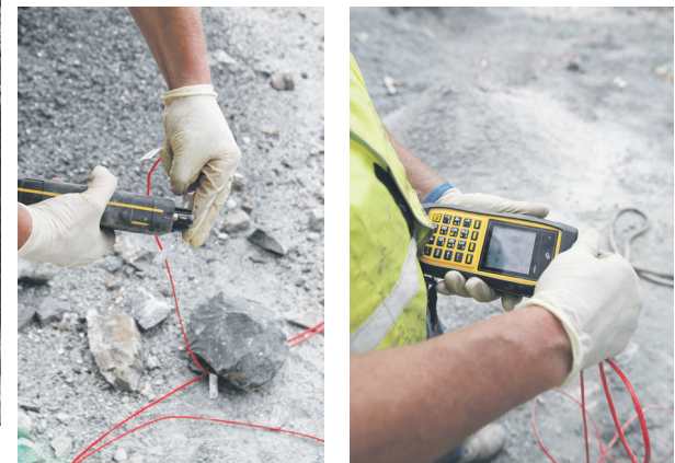
The Blaster uses a tagging unit to assign a timing sequence to each electronic detonator loaded at the Aggregate Industries — Littleton, MA Quarry.
