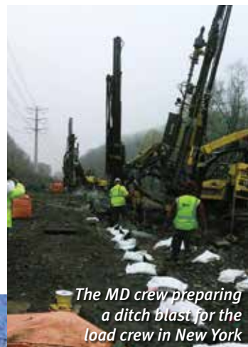
Drilling 25 feet off a hot line in New York.
